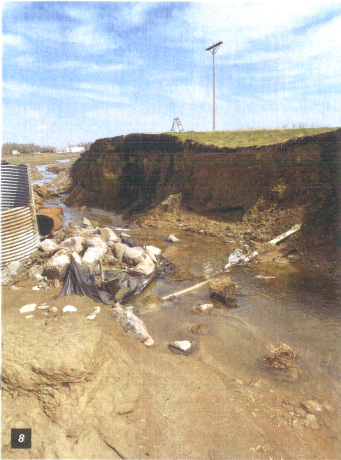
8. Wash out this spring exposed our water main.
