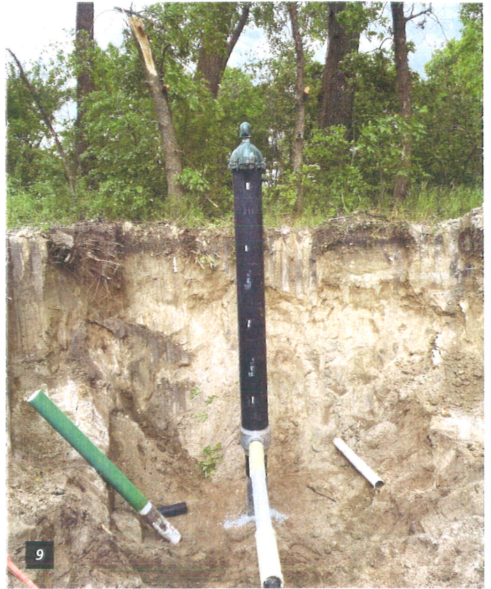
8. Wash out this spring exposed our water main.
