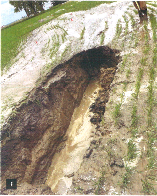
1. Raw water line leak washed all the dirt out.
