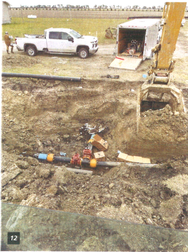
12. Tie-in to the City of Climax.
